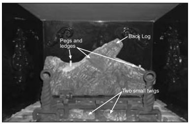
Figure 39: First Stage Log Set Installation.
